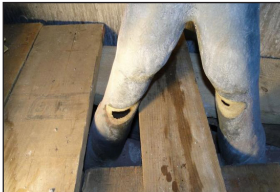
Worn section of spray header pipes
